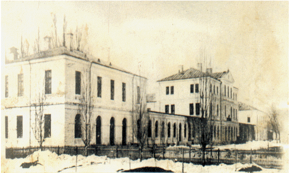
The building of the first Signal Corps Officer Candidate School Cotroceni – București
