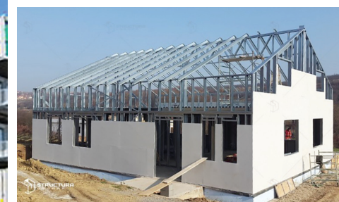
Photo 6: Lightweight construction with prefabricated structure ( https://structurausoara.ro/proiecte )
