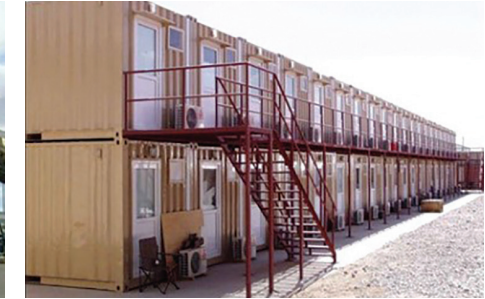
Photo 10: Modular buildings from ISO containers (DoDI 4165.56, Relocatable Facilities)
