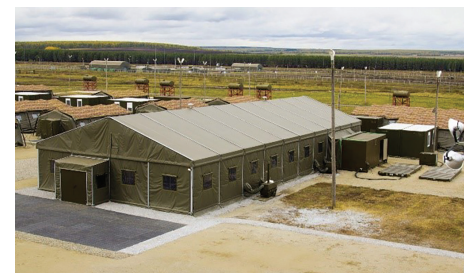
Photo 3: Tent with windfang and electrical installation ( https://ccsm.ro )
