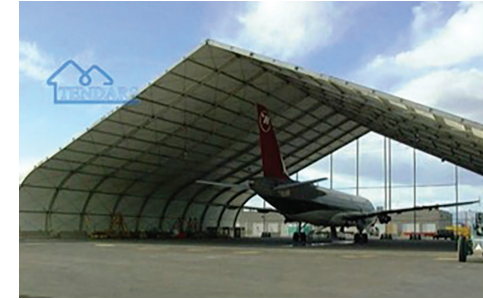
Photo 9: Textile structures with supporting framework ( http://ro.tendars-marquee.com/marquee-tent/hangar-tent.html )
