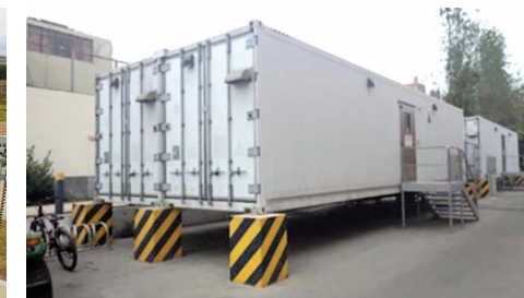
Photo 4: Container construction with temporary foundations 2
