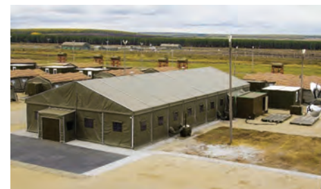
Photo 3: Tent with windfang and electrical installation ( https://ccsm.ro )
