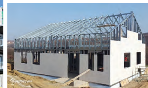
Photo 6: Lightweight construction with prefabricated structure ( https://structurausoara.ro/proiecte )
