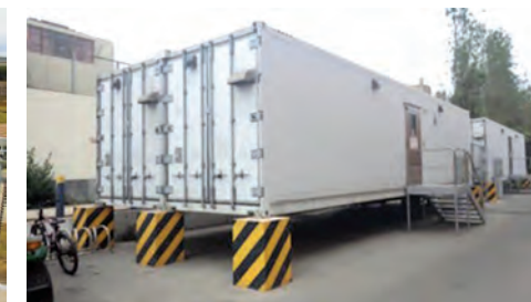
Photo 4: Container construction with temporary foundations 2
