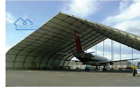
Photo 9: Textile structures with supporting framework ( http://ro.tendars-marquee.com/marquee-tent/hangar-tent.html )
